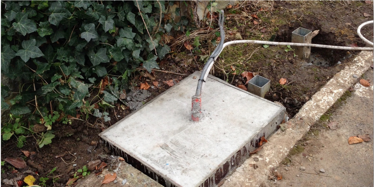
Figure 5: example of pedestal preparation with incoming power and data cables
