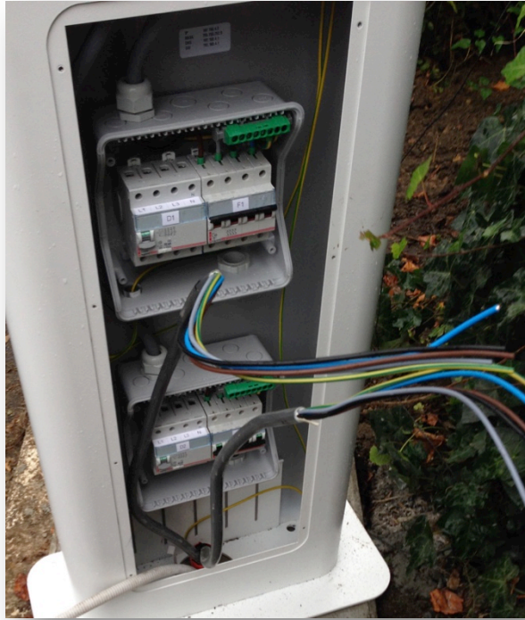
Figure 7: example of preparing the cables with open panelboard
